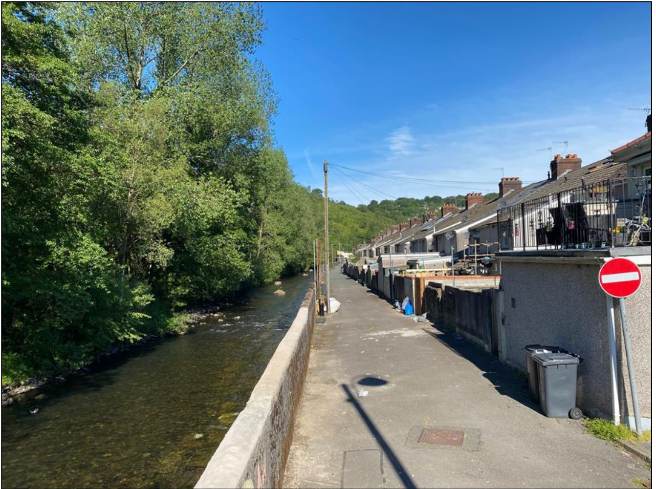
Photograph 8 Rear of Meadow Street along the bank of the River Ebbw. NRW's flood defence wall protected the street from fluvial flooding. View West. (June 2021).
