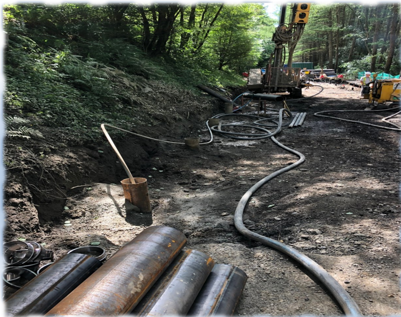
Piling works to support the proposed reinforced concrete carriageway
